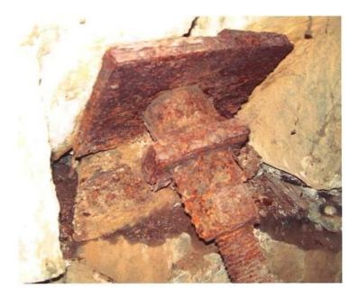
Severely corroded surface-mounted gudgeon anchor.
