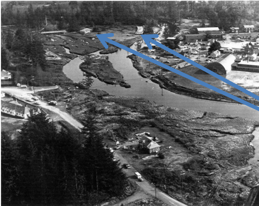
1964 Cannon Beach Bridge hit by tsunami from Alaska
