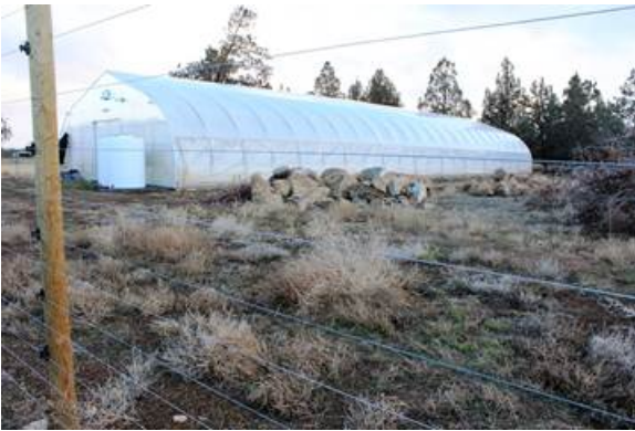
On 20 acre parcel, greenhouse is 35' from property line, neighboring existing house was already located <150' to same property line
