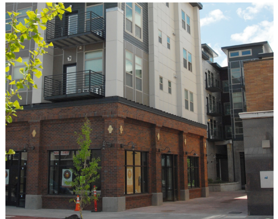
After redevelopment. The former bank building is to the right.
