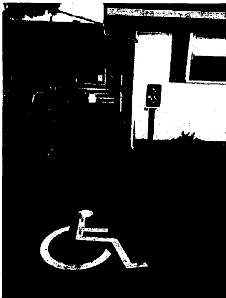
Below: Handicap parking, ramp, and entrance. This door enters through one of the exam rooms for medical. Serves all patients regardless of specialty they are seeing.
