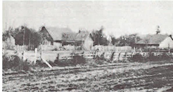
Manson House and Barn at Champoeg
