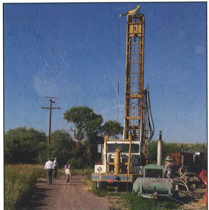
Klamath County drilled a new injection well for geothermal heated water that heated Henley High School. The project was paid in part with Recovery Act (stimulus) funds.
