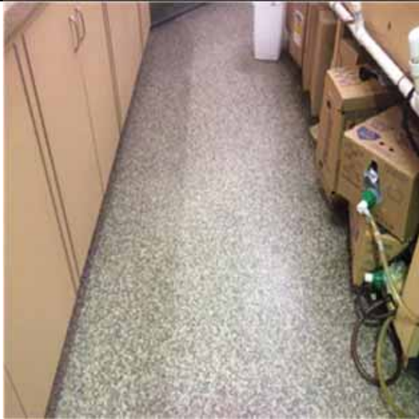
C3024 Flooring.2:- View of typical vinyl sheet.
