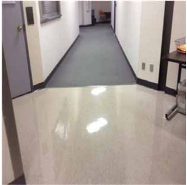
C3024 Flooring.1:- View of typical vinyl tiles.
