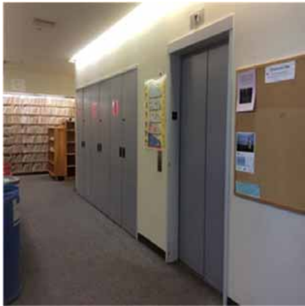
C1021 Interior Doors.3:- View of typical double hollow metal doors.
