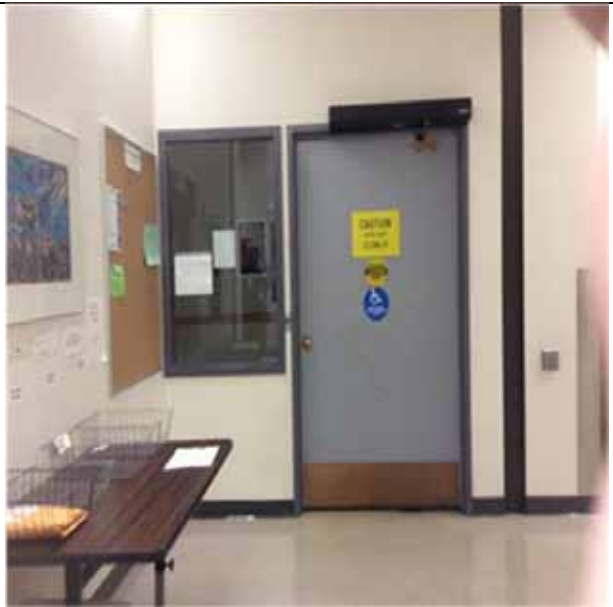
C1021 Interior Doors.2:- View of typical single hollow metal door.
