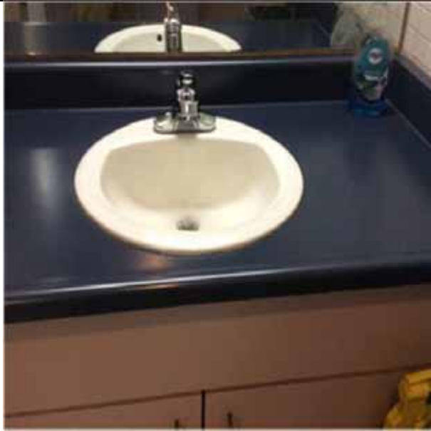
D2013 Lavatories.2:- View of one of the vanity counter top lavatories.
