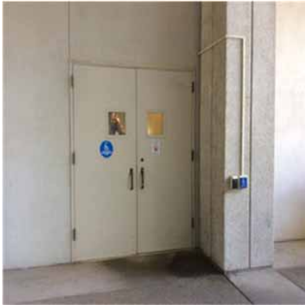
B2039 Other Doors & Entrances.2:- View of typical double hollow metal doors.
