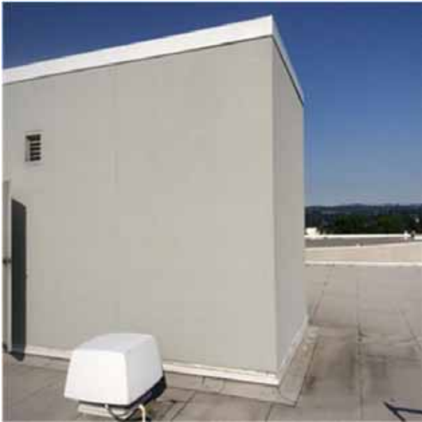
B2011 Exterior Wall Construction.2:- View of typical stucco over stud walls.
