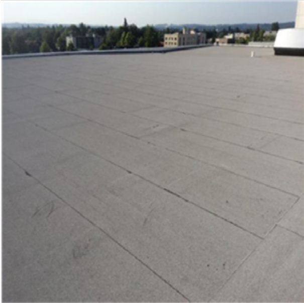
B3011 Roof Finishes.2:- View of typical built-up roof covering.
