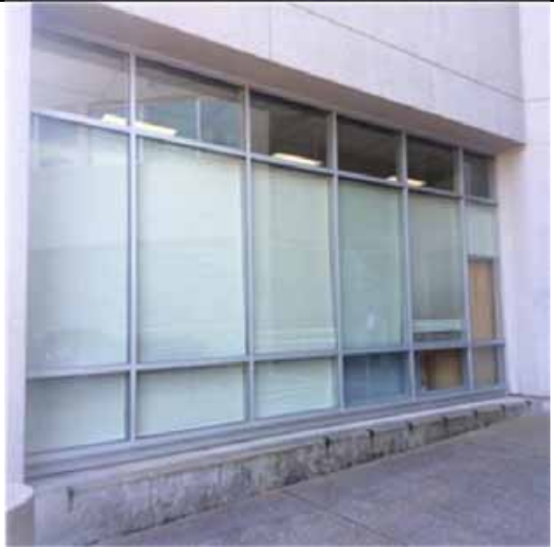
B2023 Storefronts.1:- View of typical glazed metal framed windows.
