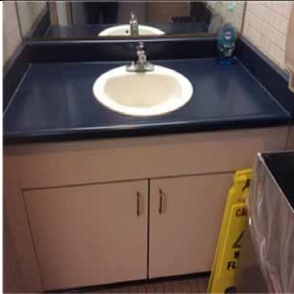
E2012 Fixed Casework.1:- View of typical floor mounted base cabinet with laminate counter top.
