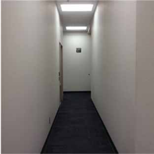
C3012 Wall Finishes to Interior Walls.1:- View of typical painted walls.
