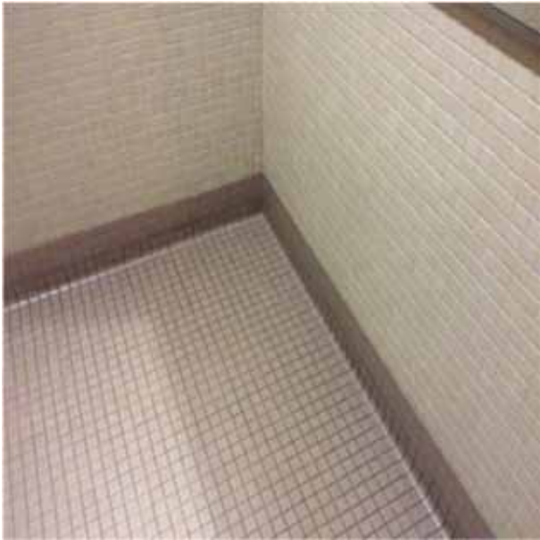
C3024 Flooring.1:- View of typical ceramic floor tiles.
