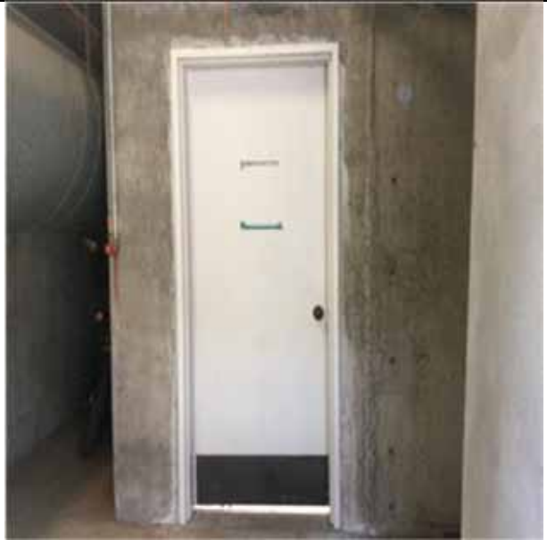
B2039 Other Doors & Entrances.1:- View of typical single hollow metal door.
