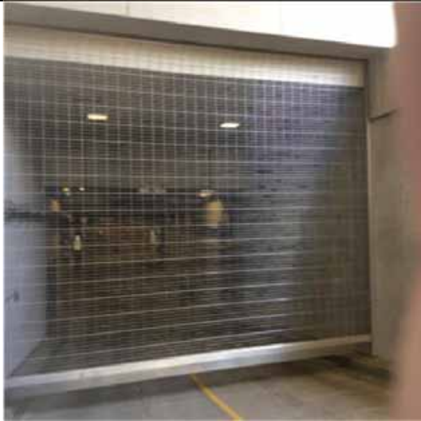
B2034 Overhead Doors.1:- View of rolling overhead door.
