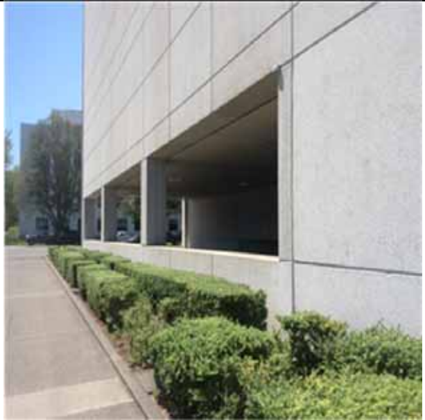
B2011 Exterior Wall Construction.1:- View of typical precast concrete walls.
