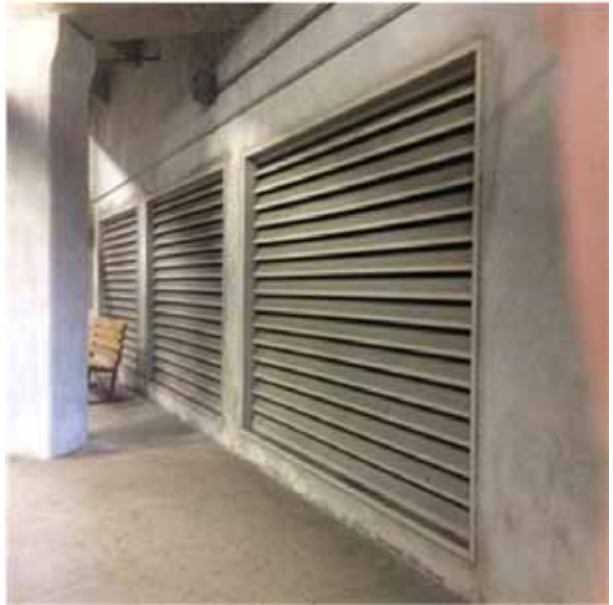
B2013 Exterior Louvers, Screens, and Fencing.1:- View of typical metal louvers.
