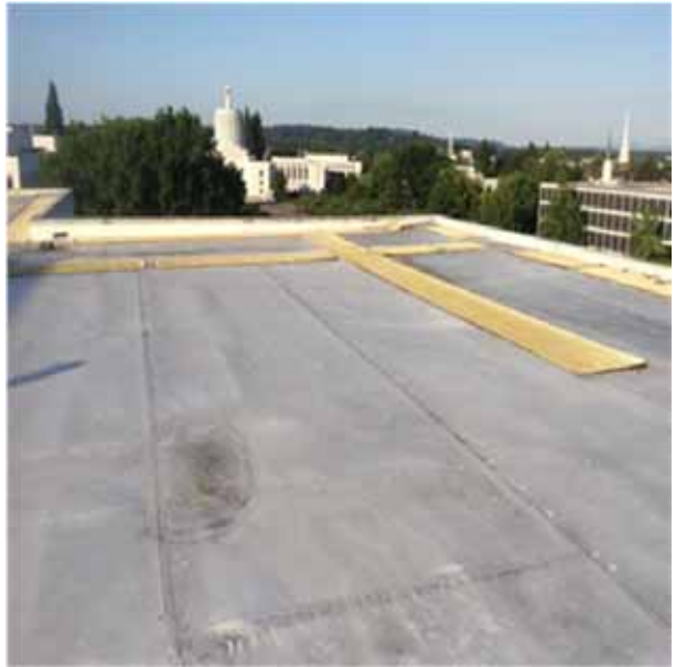
B3011 Roof Finishes.1:- View of typical TPO single-ply membrane,
