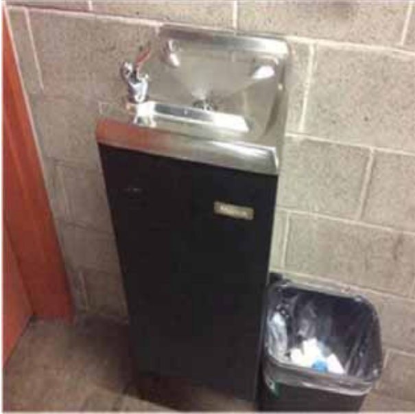
D2018 Drinking Fountains and Coolers.2:- View of the floor mounted drinking fountain.
