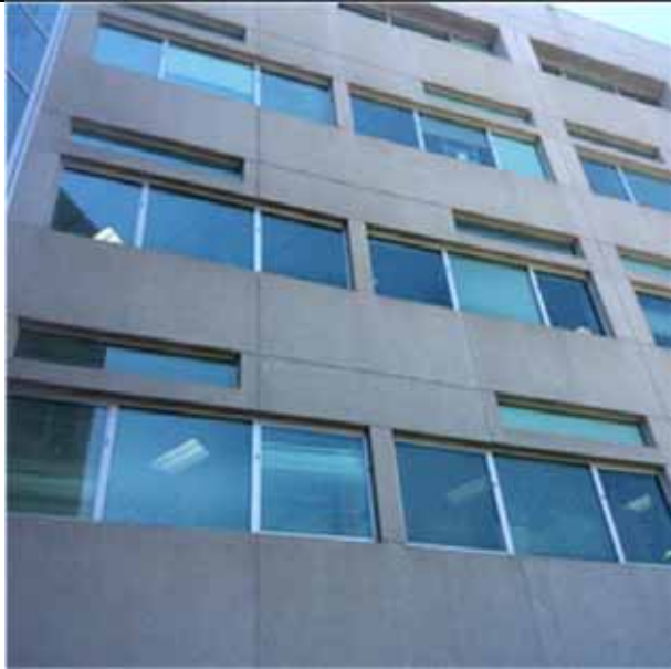
B2021 Windows.1:- View of typical aluminum window units.
