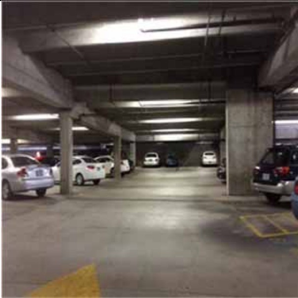
A1032 Structural Slab on Grade.1:- View of typical slab-on-grade concrete.
