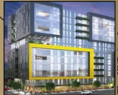
The HUB (under construction)
