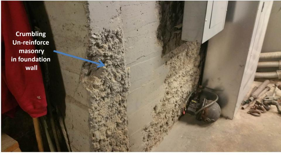
Foundation Wall of un-reinforced masonry of courthouse
