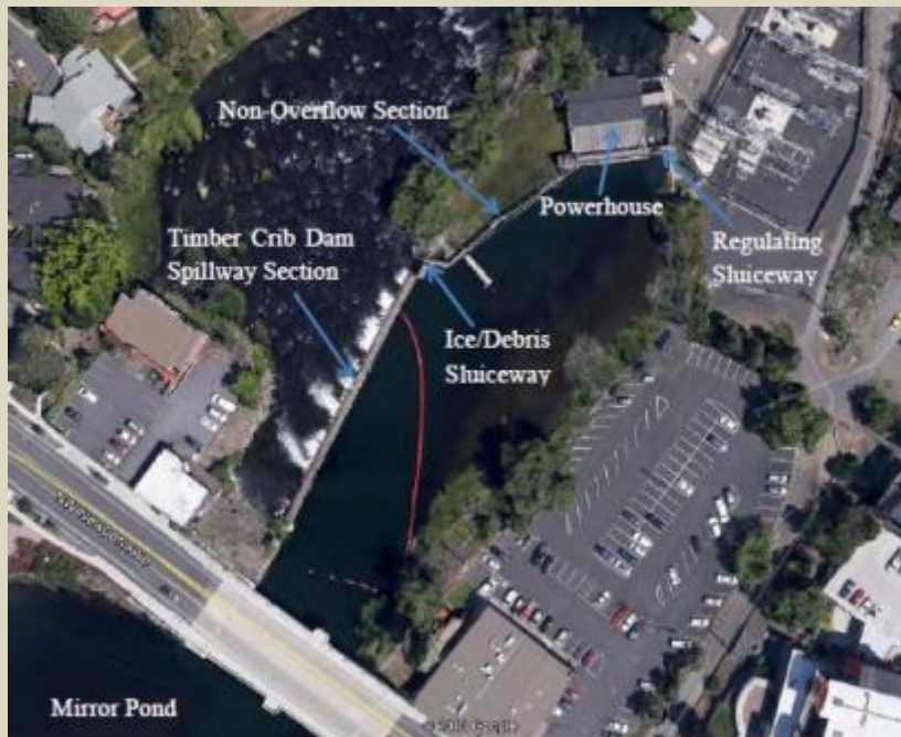
Image from Gannett Fleming dam inspection report – 05/02/2014
