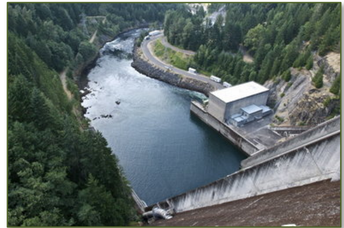
Detroit Lake Dam
