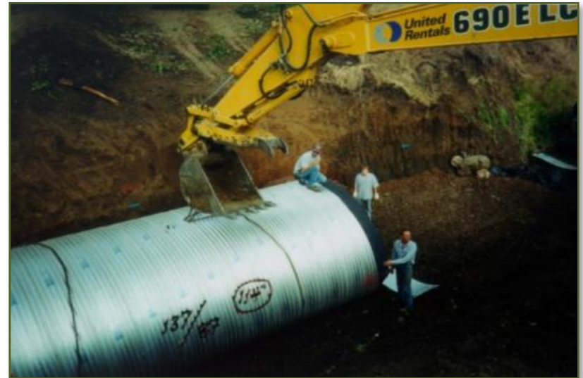
Culvert replaced to benefit fish
