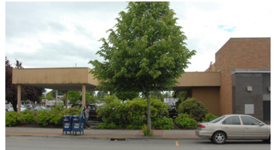
The former Wells Fargo Bank building before redevelopment.
