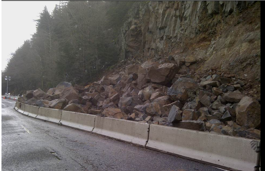
I-84 Rockfall Emergency work
