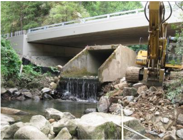
Charlotte Creek, Umpqua River: Replaced culvert with bridge and opened up 2 miles of fish habitat.
