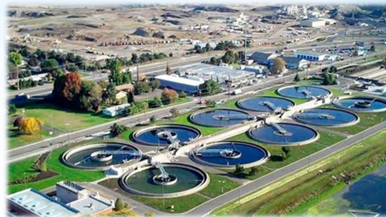
Wastewater treatment facility - Eugene, OR
