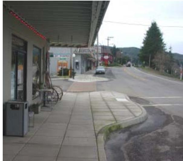
This sidewalk bulb-out in Wheeler narrows the Highway 101 crossing.
