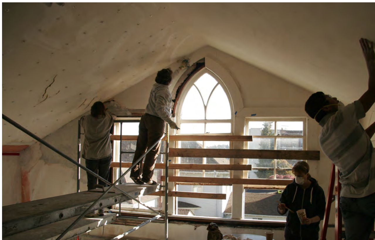
Clatsop Community College students learn how to restore historic plaster.
