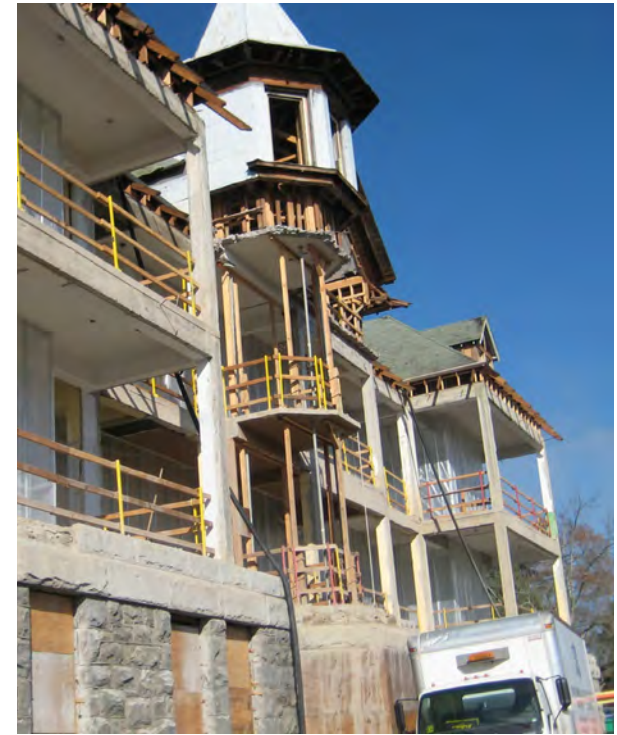
Construction on Furman Hall, Oregon State University.
