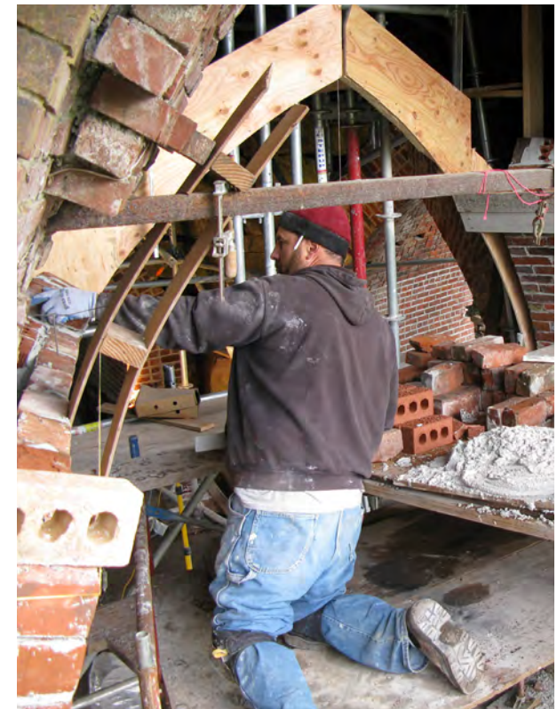
Restoring the historic arch in Lake Oswego's Iron Works.
