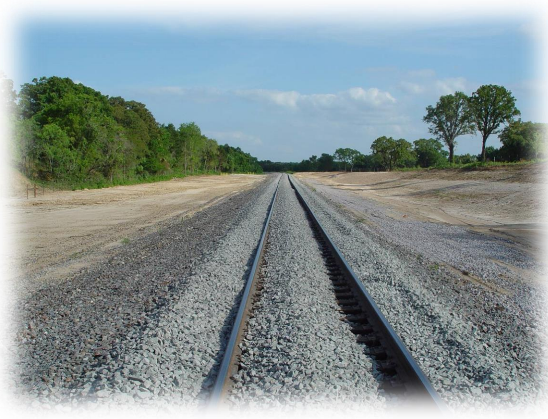
Cameron, Texas, post derailment
