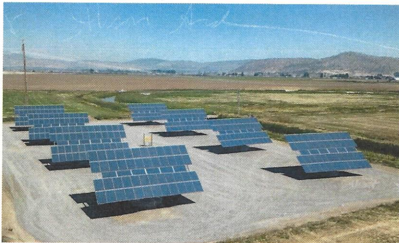
100kW Grid-Tied Tracker OSIP Installation, 2011.
