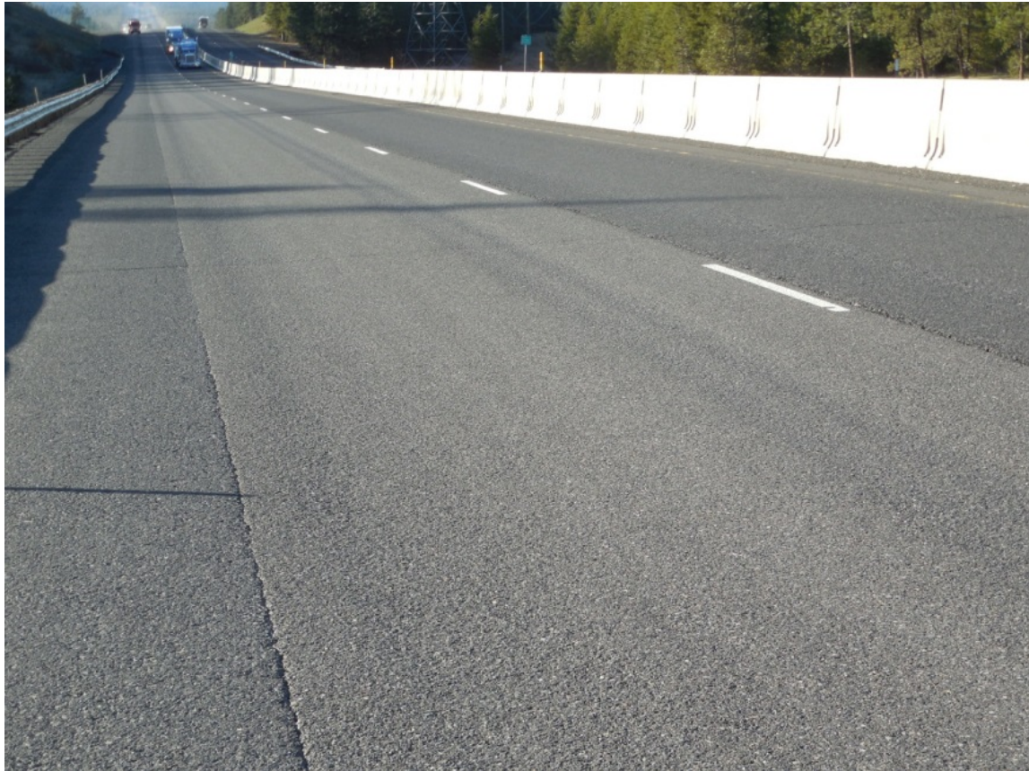
Ruts from heavy trucks—notice the 'W' shape.
