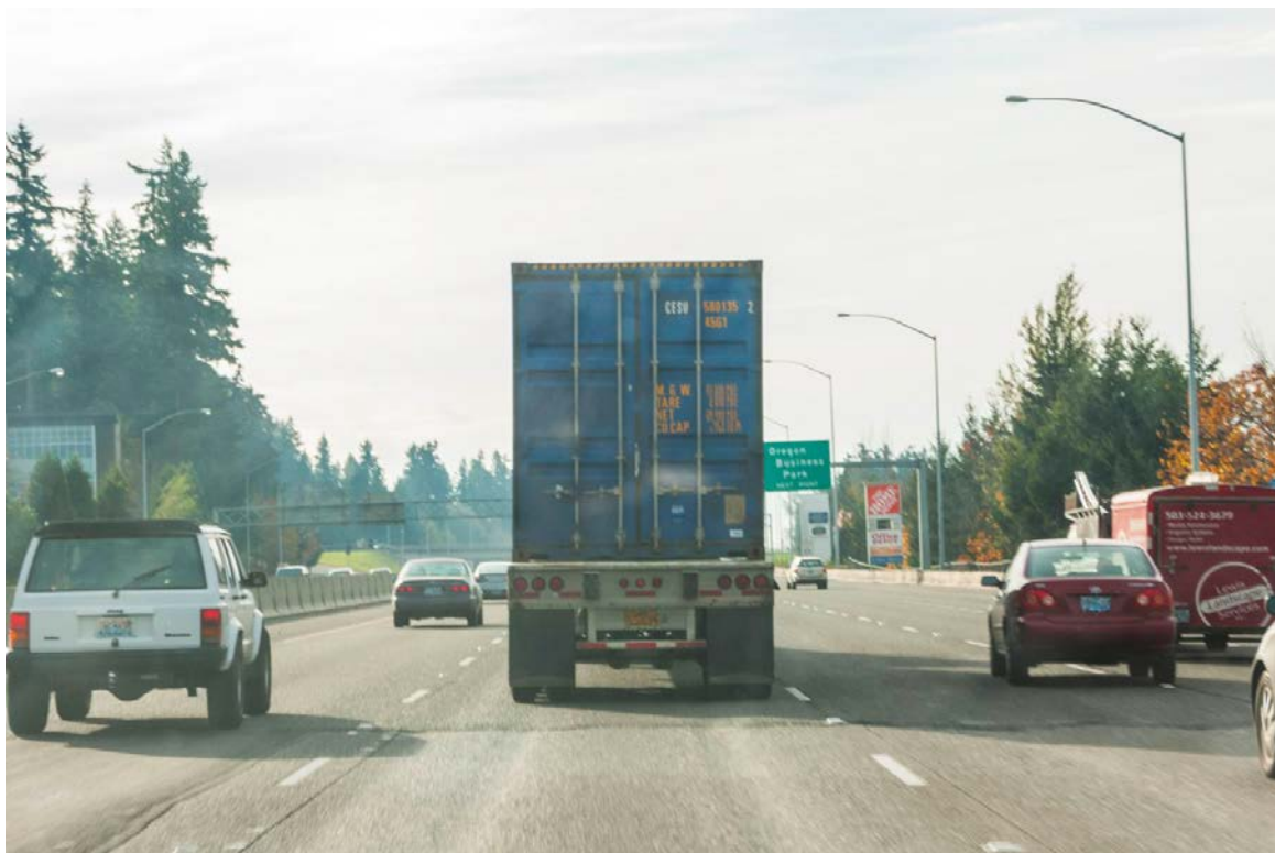
Ruts from studded tires—notice how the wheels of the truck do not align with the ruts.
