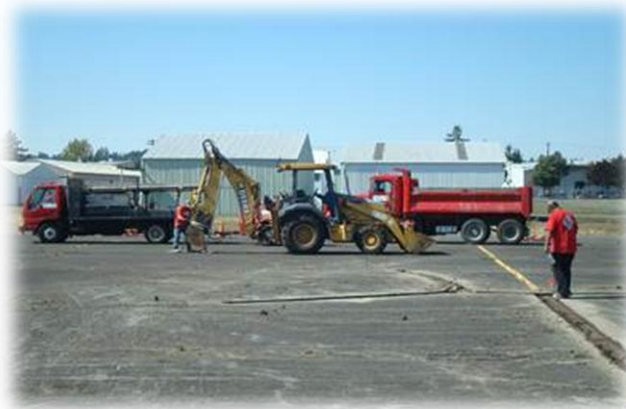
Crack sealing at Scappoose Photo credit: James Kirby, Jr., PE
