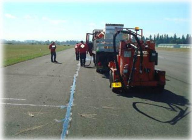
Crack sealing at Scappoose Photo credit: James Kirby, Jr., PE
