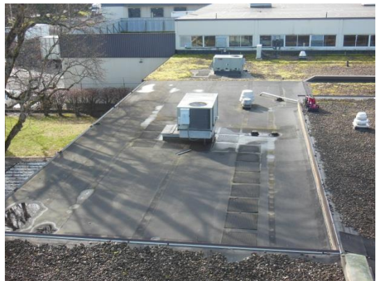
Overview of Roof Area H.
