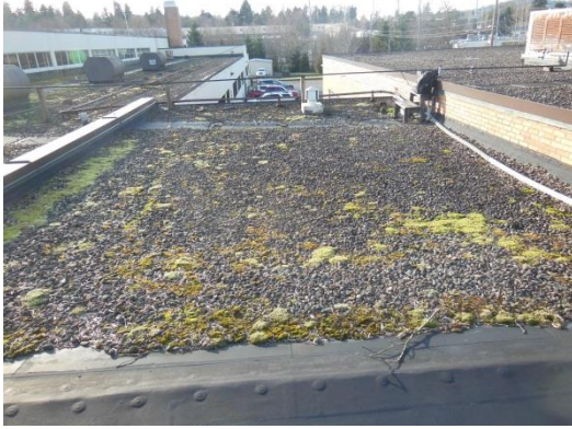
Overview of Roof Area I looking west.
