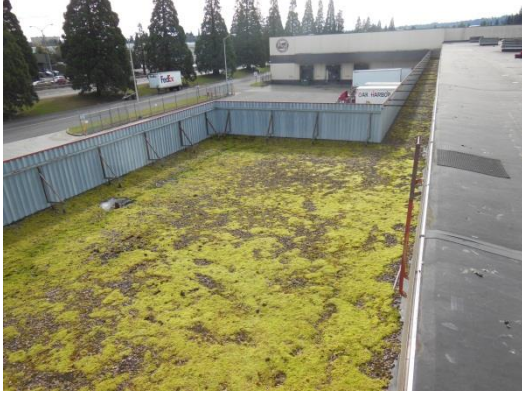
Overview of Roof Area D looking south.
