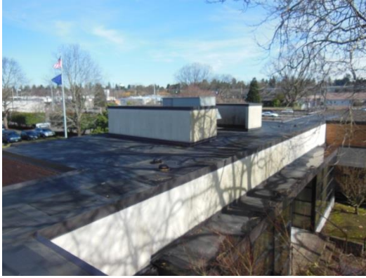
Overview of Roof Area P.
