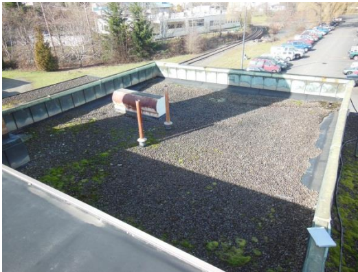
Overview of Roof Area F.
