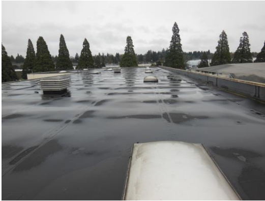
Overview of Roof Area A.
