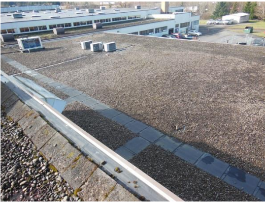
Overview of Roof Area K looking south.
