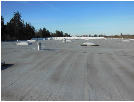
Overview of the roof surface looking north.
