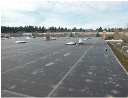
Overview of Roof Area C looking west.
