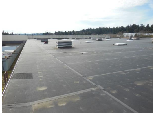
Overview of Roof Area C looking south.
