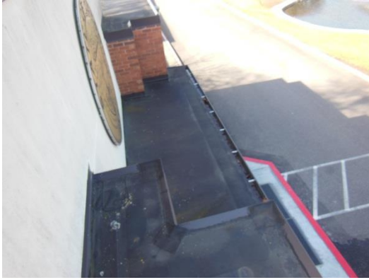
Overview of Roof Area R.
