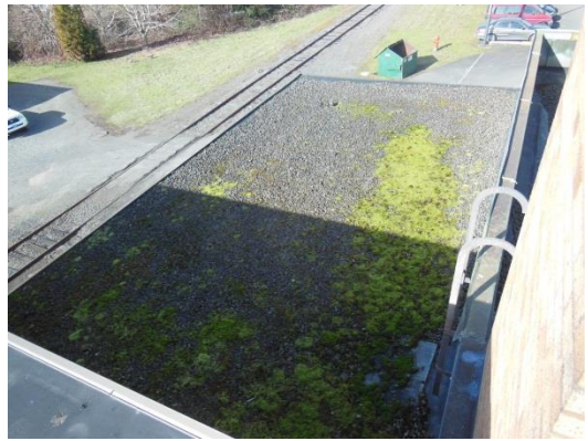
Overview of Roof Area G.
