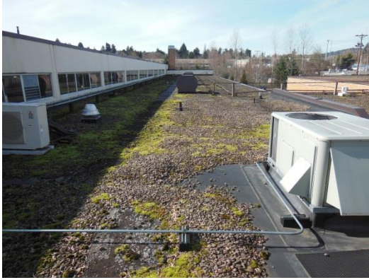
Overview of Roof Area E looking west.
