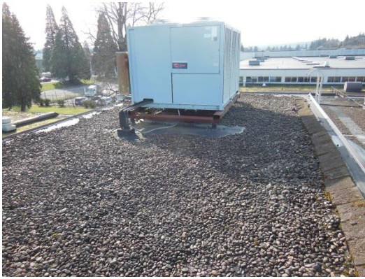
Overview of Roof Area L.
