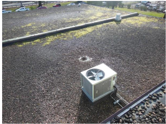
Overview of Roof Area M.
