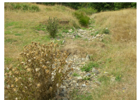
After photo one year after treatment (same as above), note the vegetation reestablishing within the rock plug
