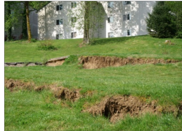
(top) New lidar-based landslide inventory map of the Oregon City area. The red landslides are ones that have moved historically. Many of these caused significant damage to residential homes and apartments (bottom). Photo is the first ground cracks at the Newell Creek Apartments in 2005. After two years of movement, many of the buildings were severely damaged and had to be condemned and demolished.
