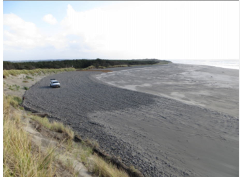
The USACE revetment involved placement of gravel along the shore to prevent continued erosion of the beach and threats to the jetty.
