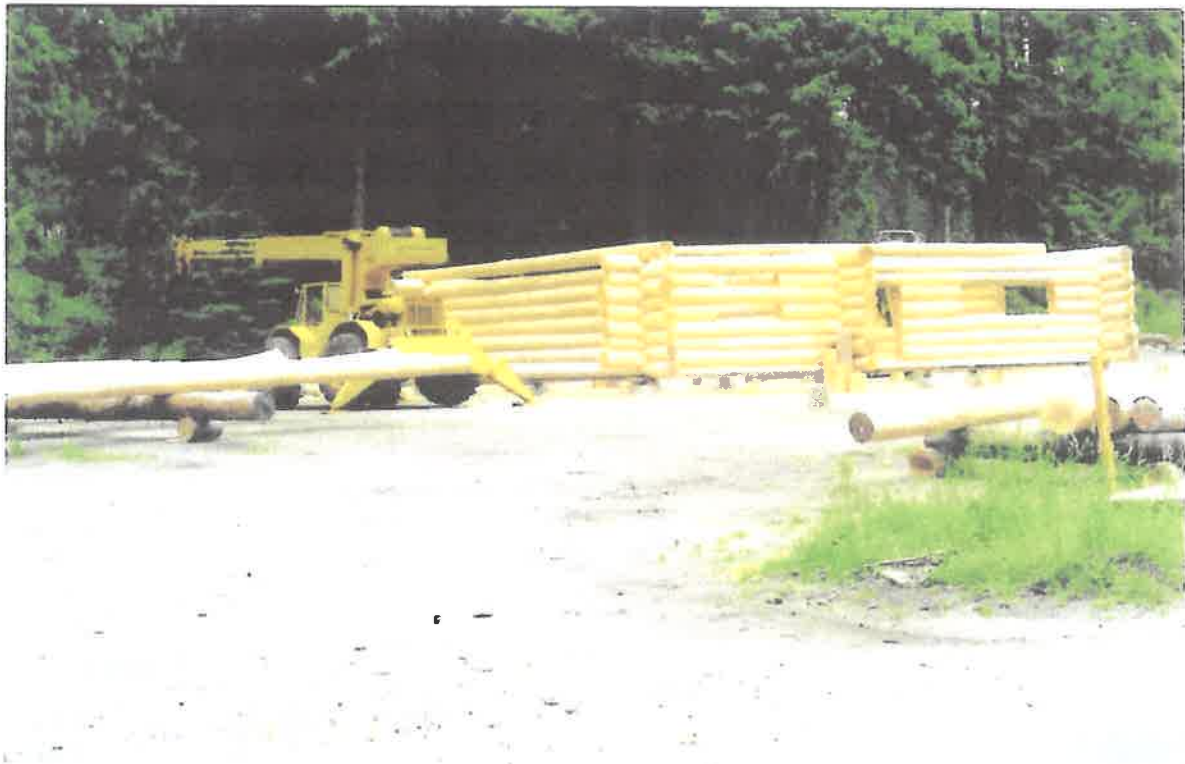
View of home-manufacturing and construction work area along E. Marmot Road (foreground) and heavy equipment routinely used and operated.
