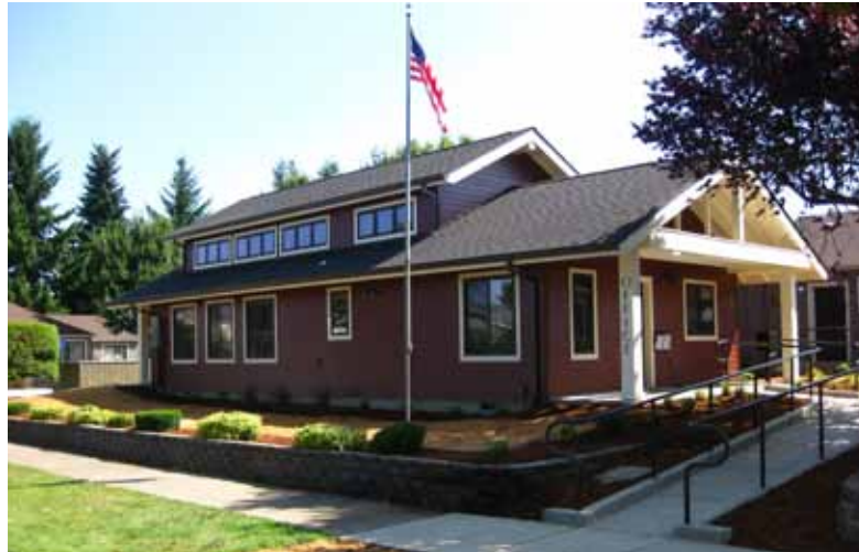
The Village Apartments were extensively remodeled using Housing Preservation Funds provided by Oregon Housing and Community Services.
