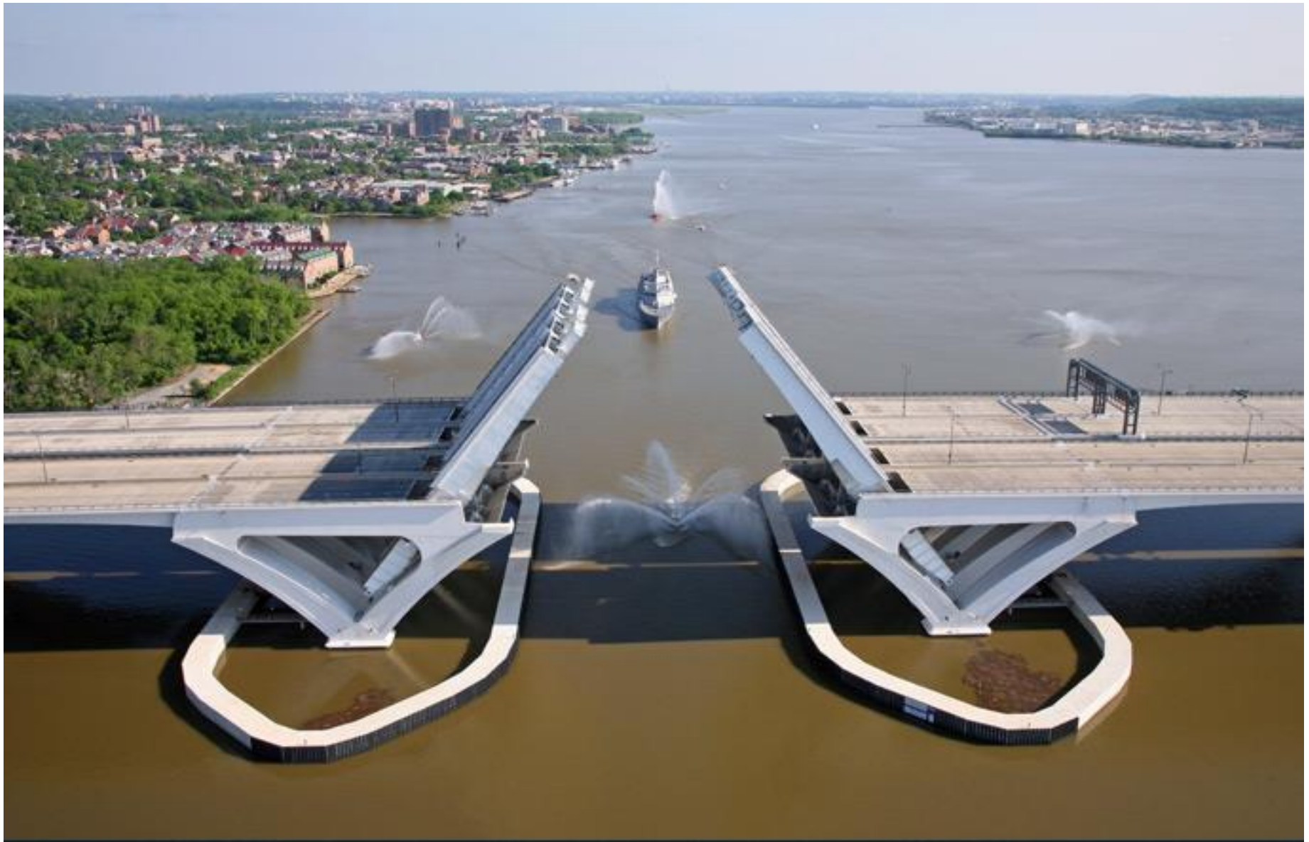
Bascule draw span similar to this new Woodrow Wilson I-95 Bridge in Washington DC
