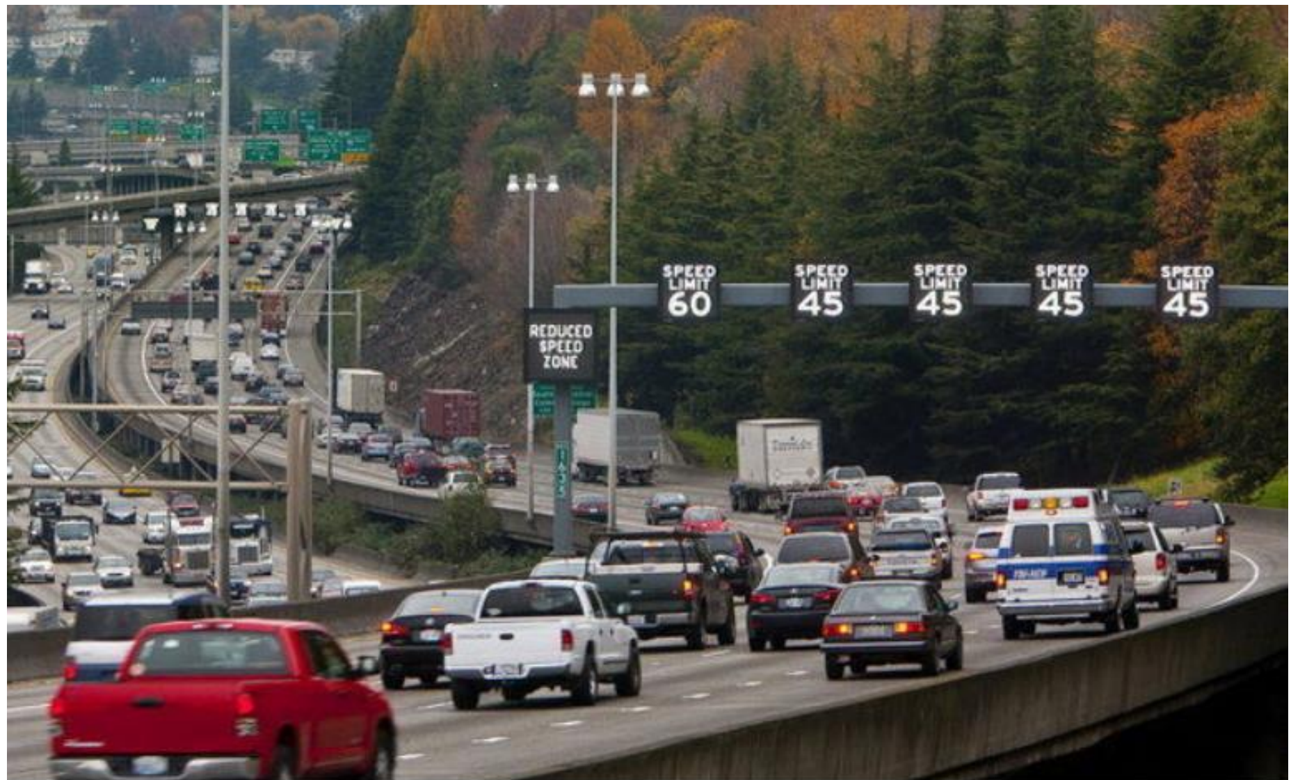
Variable speed-limit signs stare down at drivers heading north along Interstate 5 in the Seattle area. The signs, coming soon to Portland, are intended to help improve the flow of the commute. (Mike Siegel/Seattle Times)
