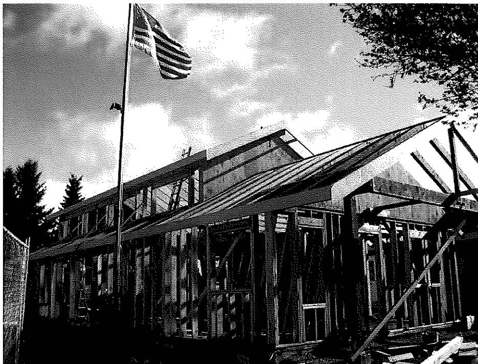
The Village Apartments were extensively remodeled using Housing Preservation Funds provided by Oregon Housing and Community Services.
