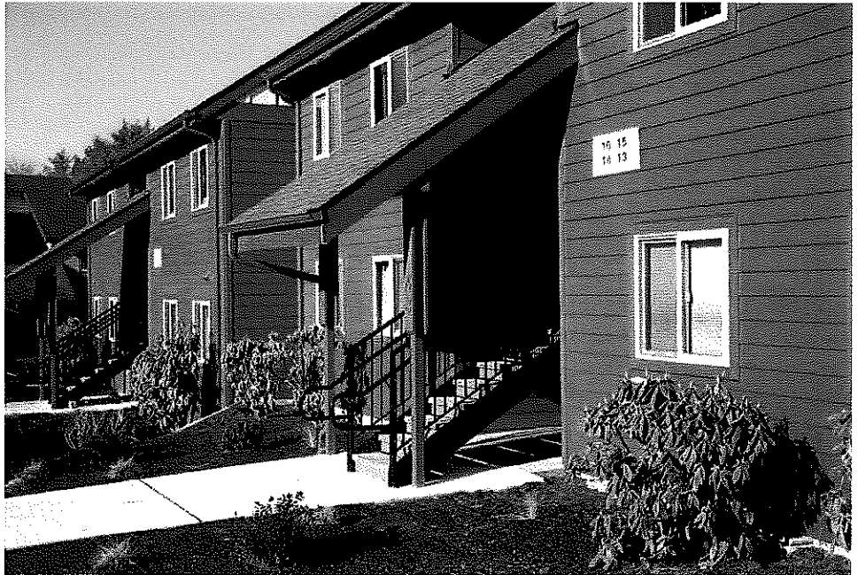
The Spyglass Apartments were originally built through a US Department of Agriculture (USDA) Rural Development program. The aging complex has been given new life with much-needed renovations.
