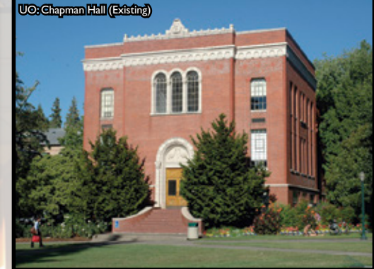
UO: Chapman Hall (Existing)
