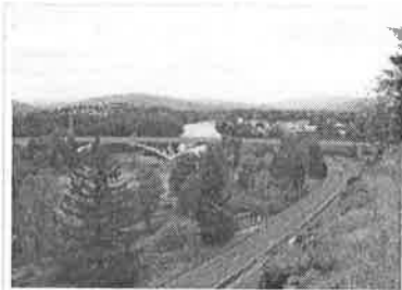
The Willamette River Bridge in Eugene was one of 477 bridges that fit the criteria to be labeled structurally deficient by ODOT engineers. The bridge is currently in the process of being repaired and is expected to be open to traffic by 2013. (Rendering courtesy of ODOT)
