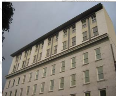
The Estate – renovation completed in December 2007
