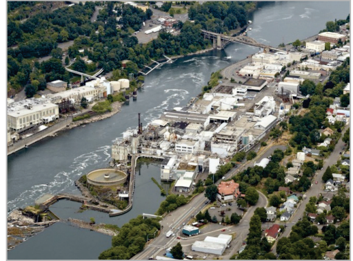
Former Blue Heron Paper Co. along the Willamette River
