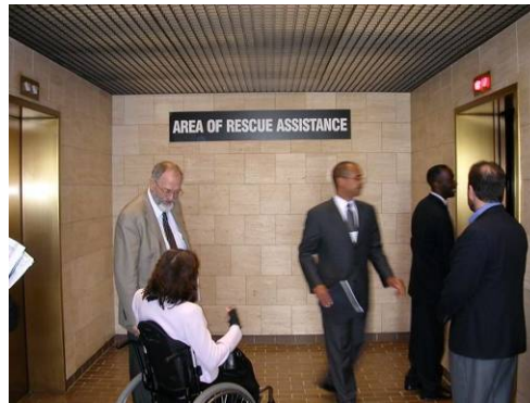
Figure: Designated area of refuge next to elevators
