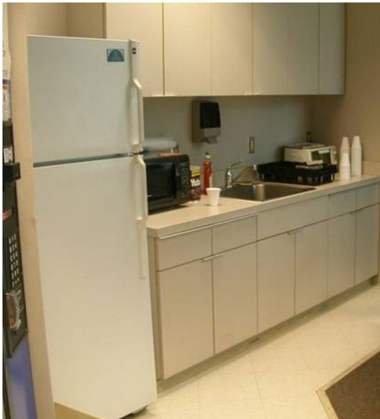
Figure: Side approach to service unit if range or cooktop not provided
