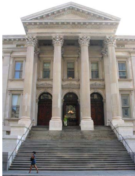
Figure: Plinth with stairs creating access problems
