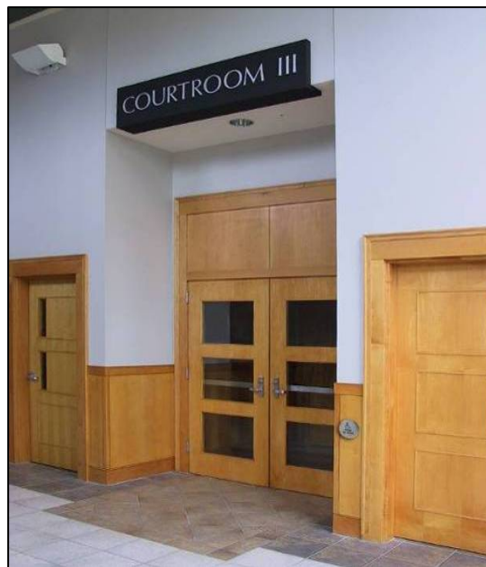
Figure: Automatic door operator with controls located outside door swing.
