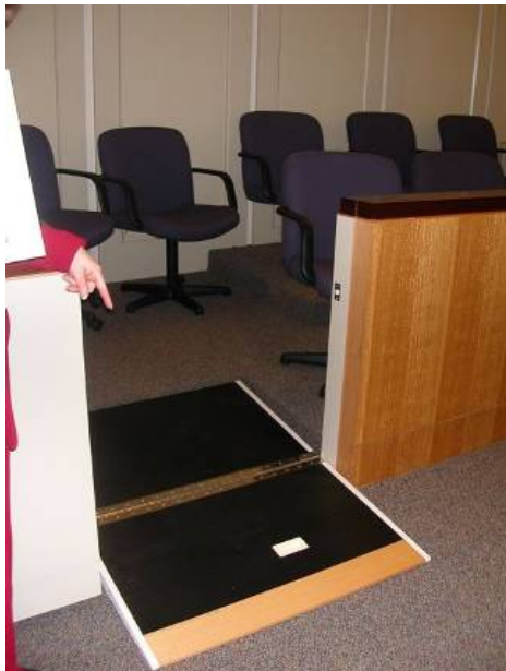
Figures: Common Error -These flip down ramps require assistance to create the accessible route, and when open, block the gate and maneuvering space for the door.
