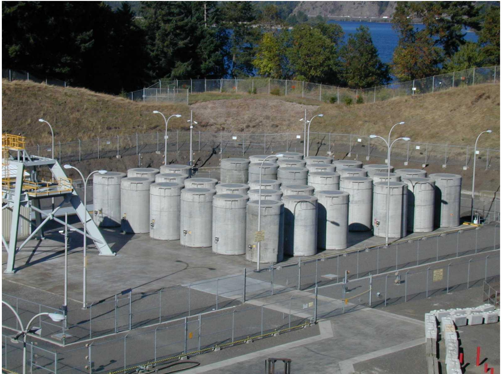
Trojan Independent Spent Fuel Storage Facility
