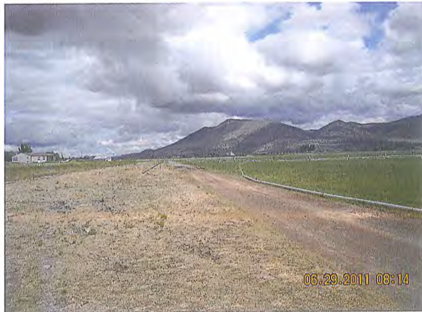
Airport Site Inspection Photo
