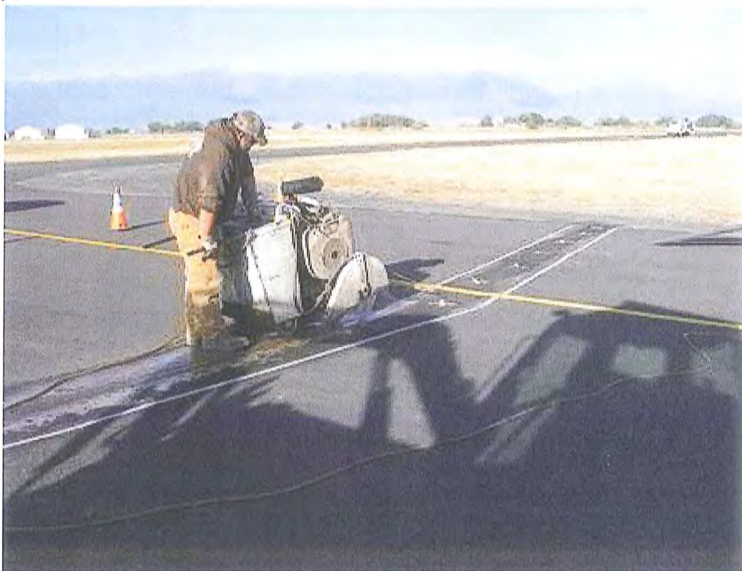
Pavement Maintenance (Crack Repair) at Baker City
