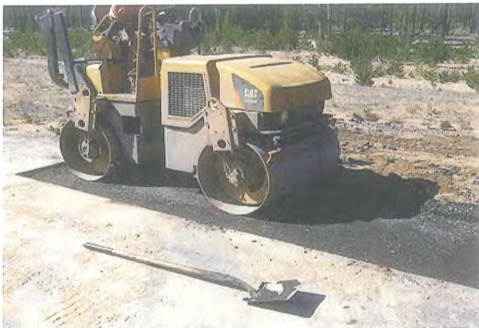
Crescent Lake Runway Repair
