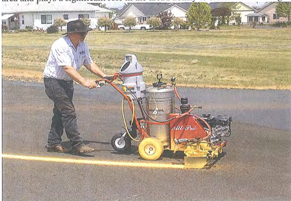
Striping Independence State Airport
