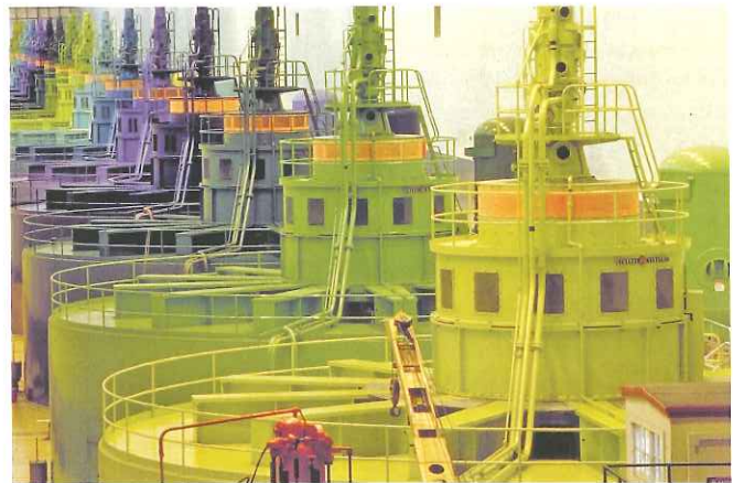
Increased hydroelectric production under the Treaty has benefitted both Canada and the United States.
