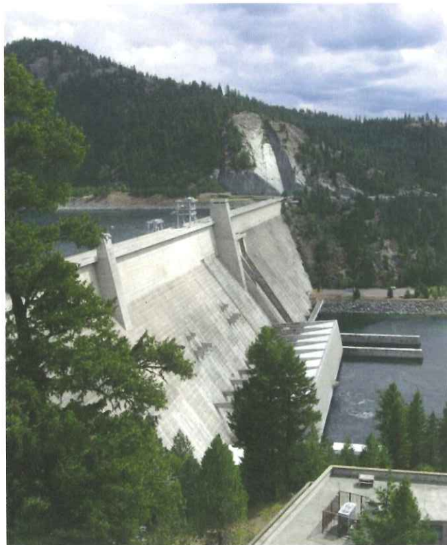
Libby Dam, the last Treaty dam to become operational is the only Treaty dam in the United States.
