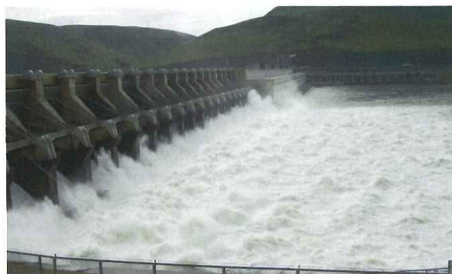
Spill helps young fish migrate past dams, but high levels increase total dissolved gas, degrading water quality.
