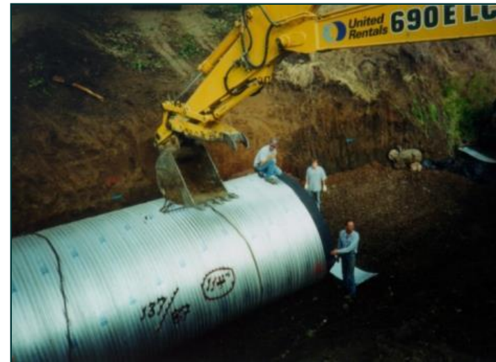
Culvert replaced to benefit fish
