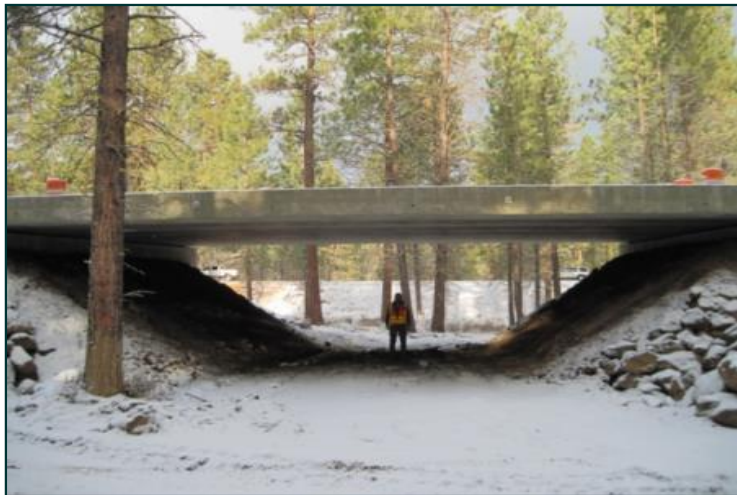
Wildlife corridor on Highway 97
