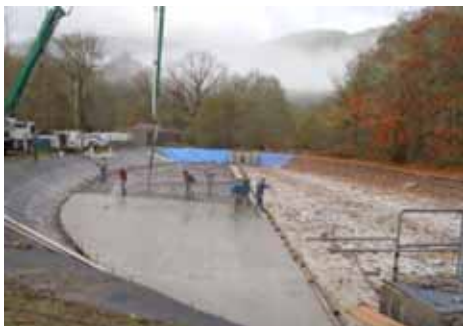
Installing new lining in Rhoades Pond.
