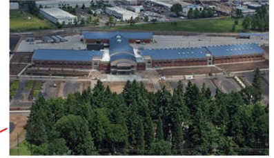
Camp Withycombe AFRC 7kW Solar
