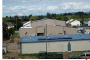
Gresham Armory 3.5kW Solar
