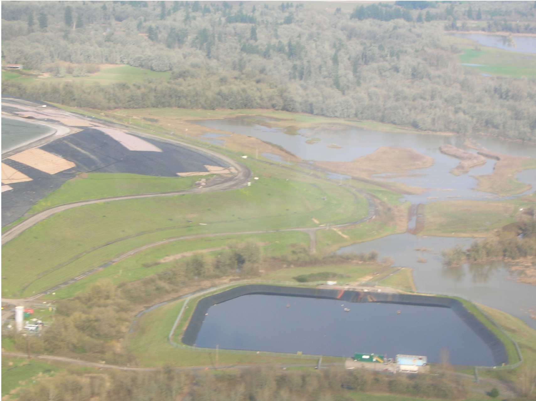
Riverbend Landfill - 2 April 2012 Looking West to East
