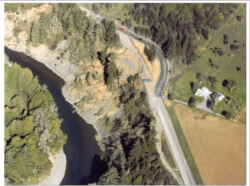
The Powers Landslide at Mile Post 14
