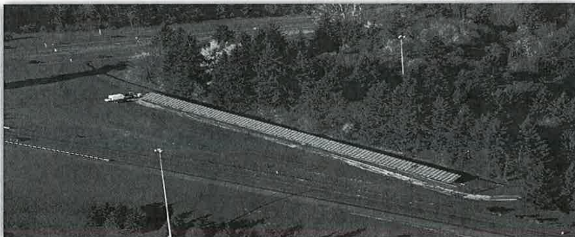
Oregon Solar Highway Pilot project at I-5 and I-205
